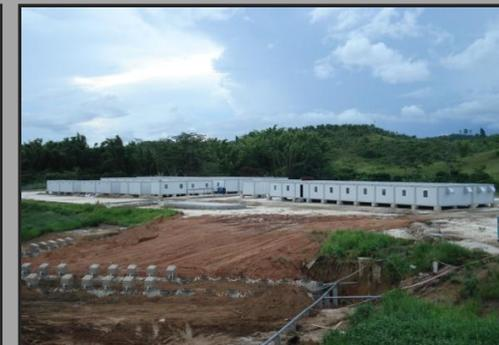
Can be erected on level concrete ground or on concrete blocks
